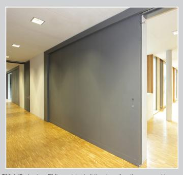
T30-1 "Teckentrup E" fire-resistant sliding door: A wall recess enables flush installation, and an artificial header was installed directly on the ceiling for the upper attachment of the floor-to-ceiling door. Counterweights and runner rails are fully encased and match the colour of the building.
