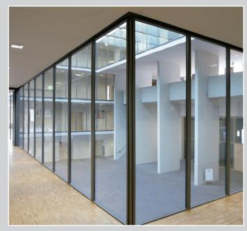
Light, Air and Openness – the foyer of the Max-Born-Kolleg is extremely spacious. The floor-to-ceiling glazing of the galleries provides both fire and fall protection in one. Due to the large panes of glass a special type of attachment had to be found that would receive building authority approval or be accepted in individual cases.
