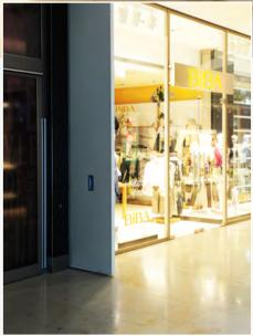
The special attraction of the elegantly hidden fire doors is the integration into the visible surface: decorative stainless steel recess traps disguise the T90 doors which are around six metres wide and four metres high. This covering has the effect of a deliberate turning point of design between the rows of shop windows. Probably only a few people will suspect that a technically necessary component is located behind them.
