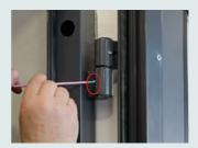
**2.** Open the door, loosen the M6x5 set screw (4mm allen key).
