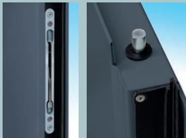
The inactive leaf is secured with flush bolts to the top and bottom of the leaf.
