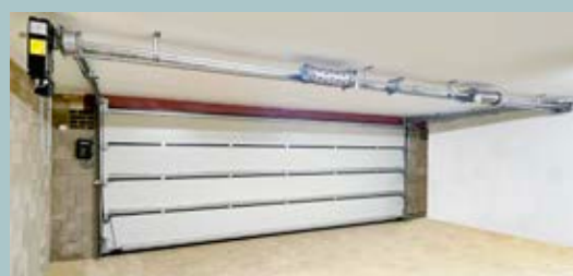
Low headroom rear torsion spring option.
