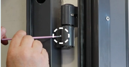
3. Open the door, loosen the M6x5 set screw (4mm allen key).
