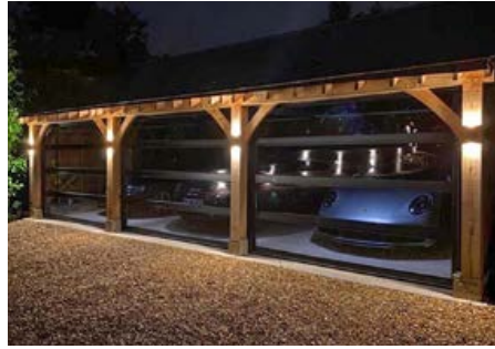
Full width glazing up to 3000mm wide (no mullions)
