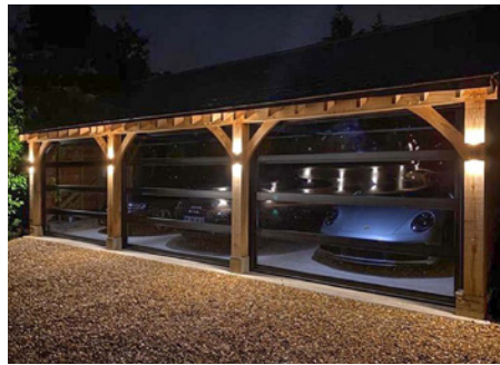
Full width glazing up to 3250mm wide (no mullions)
